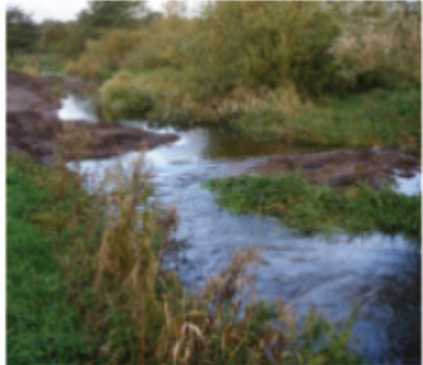
Image: Redistribution of existing gravel bed and re-profiling of spoil banks creates a narrower, more sinuous river course
