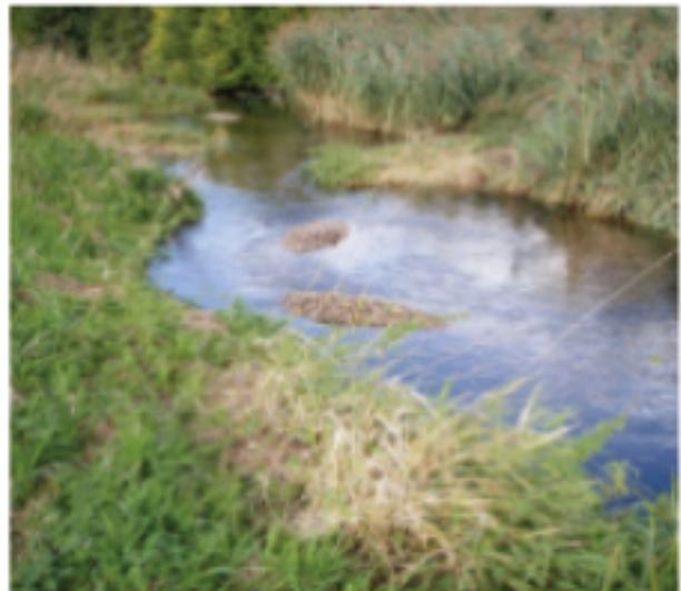
Image: Newly installed gravel glide, resulting in varying river bed height and flow diversity
