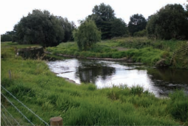
New glide, berm (opposite bank) and plug (far left) diverting flow along meander loop.
